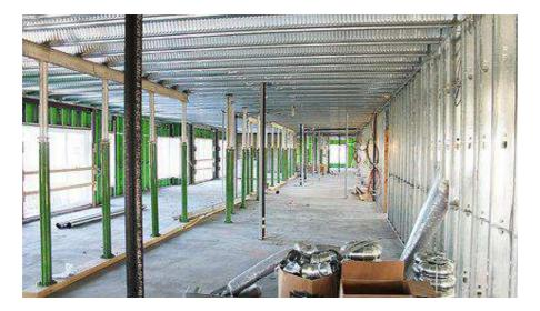
**Unshored construction** – the steel beam or steel deck supports formwork, concrete and its selfweight.
