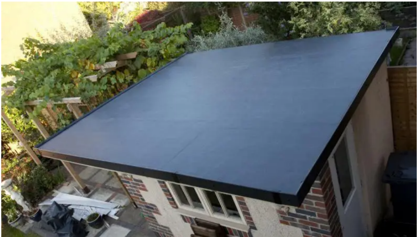
EXAMPLE OF FLAT ROOF MEMBRANE
