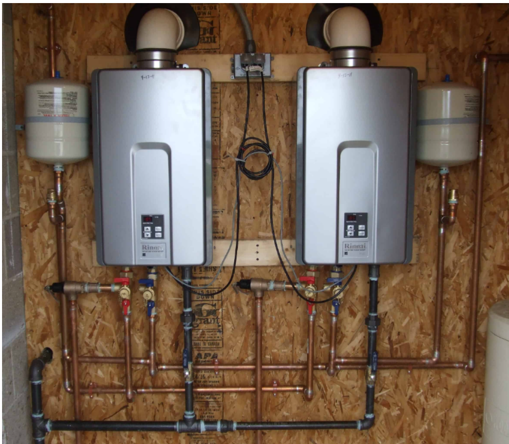
EXAMPLE ONLY: TANKLESS BOILERS (NEWER MODELS)
