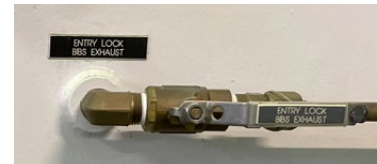
BIBS exhaust shell valve
