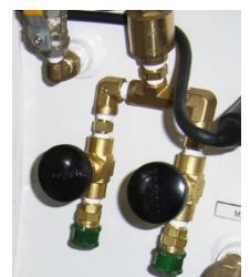
BIBS supply connections
