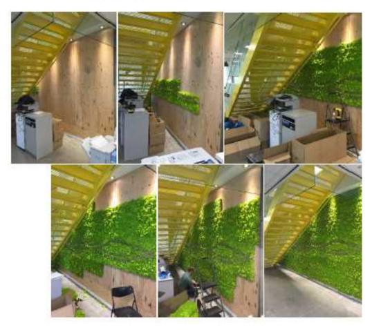
The Reindeer Moss is glued onto a sheet of Coroplast or Eco Felt (other panel options include wood, cork or flexifelt for round surfaces). Standard sized panels are 36" x 12". The Mossart panels are 1.5 lbs per sqft and can be easily installed directly onto drywall or plywood.
