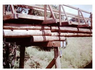
These laminated log footbridges have shear plates fitted internally on both logs where the bolts pass through. In the presenter's opinion, what is a limitation of these plates?
