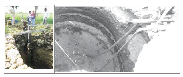
**Photo 1 and 2**. Typical wells in Bhatiya, Gujarat. "Left photo" with only engine pump fitted and "right photo" with DC pumpset installed. Note: because of the excessive well depth the pumps needed to be placed "down the well" in order to not exceed the maximum suction lift.
