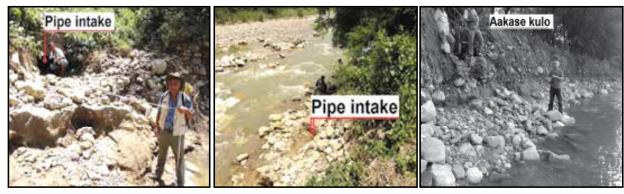
Eroded river bed at the intake of the Aakase kulo after July flood
