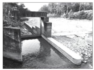
Figure 2: Permanent intake of SIS
