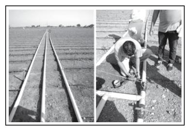
**Photo 5 & 6**. Main delivery line and submain zone lines with drip line offtakes.
