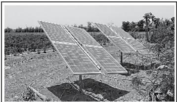
**Photo 3**. Two 400 W solar arrays each with manual tracking mounts.
