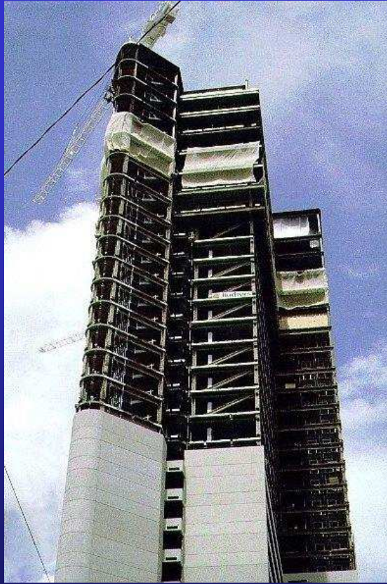
Nashville Convention Centre, tower overview
