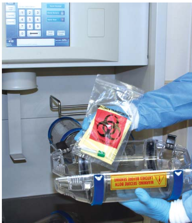
Figure 12-13 Specimen prepared for transport through pneumatic tube system.
