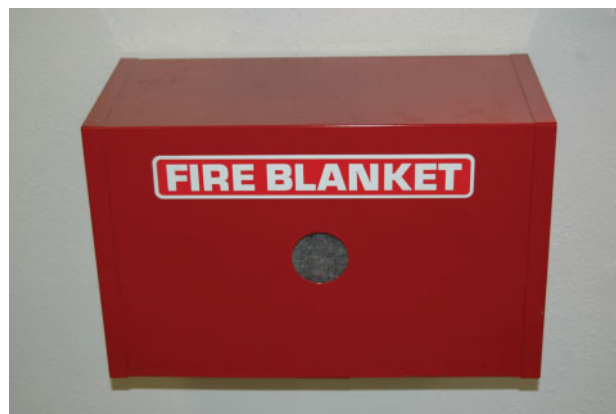
Figure 3-13 Fire blanket storage box.
