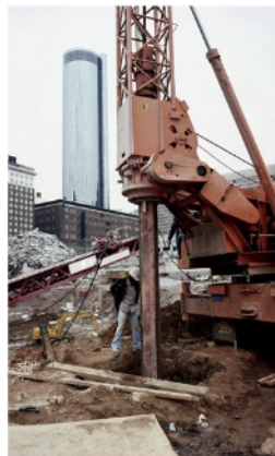
Figure 4 A pile driver in action
