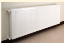
Figure 6 A central heating radiator
