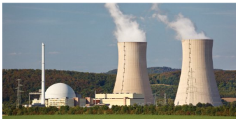
Figure 2 A nuclear power station
