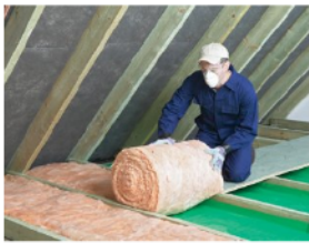
Figure 3 Insulating a loft. The air trapped between fibres make fibreglass a good insulator.
