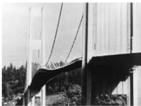
Figure 2 The Tacoma Narrows Bridge in the USA twisting just before it collapsed
