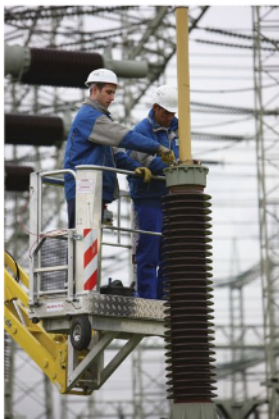
Figure 1 A power transformer under inspection
