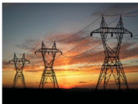
Figure 2 Electricity pylons carry the high voltage cables of the National Grid
