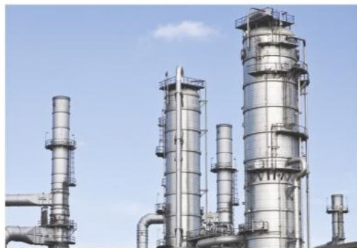
Figure 1 In an oil refinery, huge crackers like this are used to break down large hydrocarbon molecules into smaller, more useful ones. The petrochemical industry source the chemicals used to make products such as solvents, lubricants, polymers, and detergents, as well as the fuels that modern life depends on
