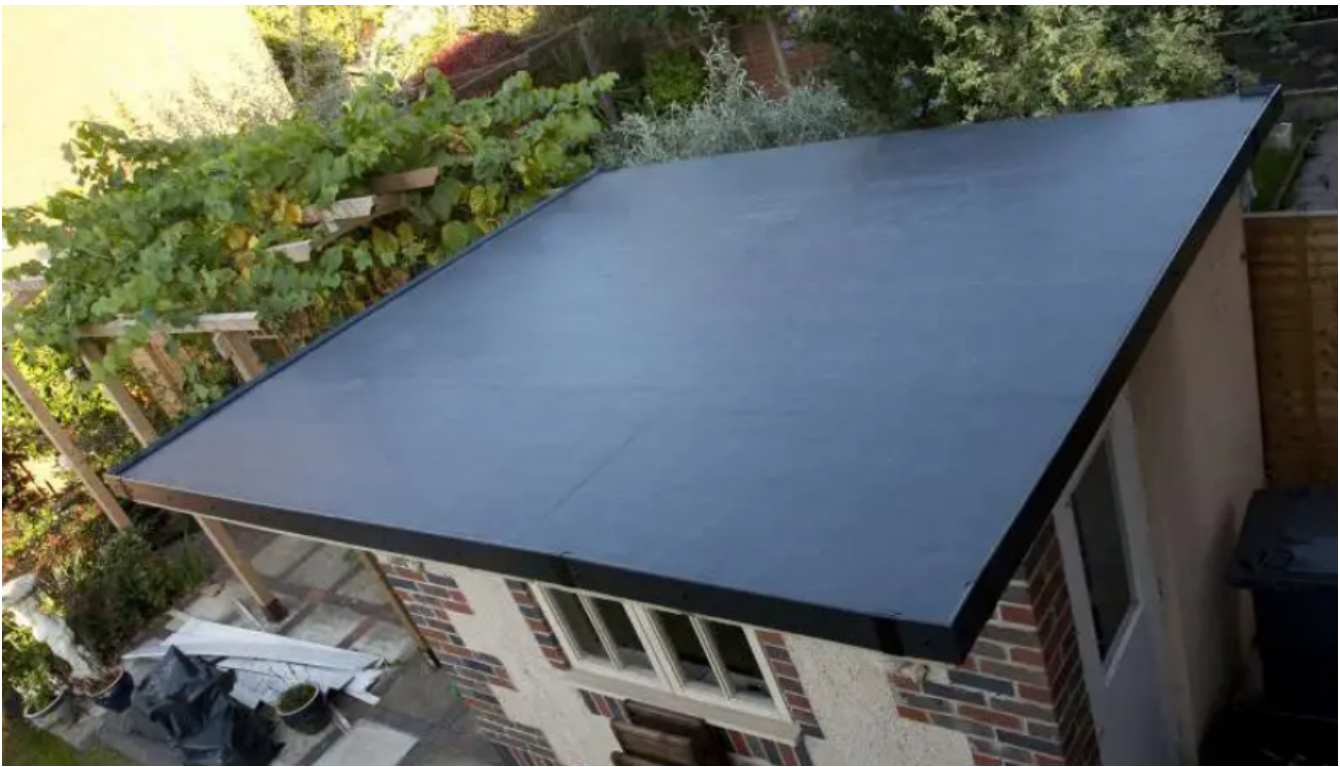
EXAMPLE OF FLAT ROOF MEMBRANE
