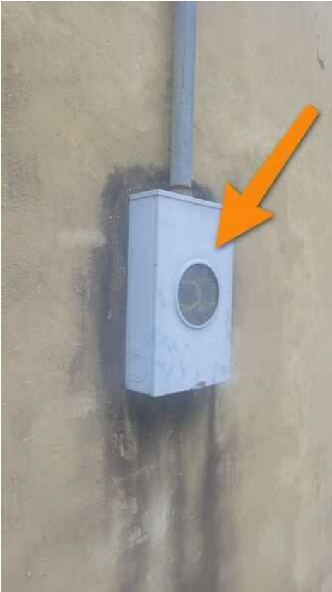
Meter pulled by the electric company
