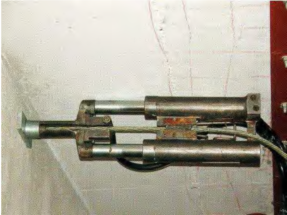
A gripper jack stressing a tendon.
