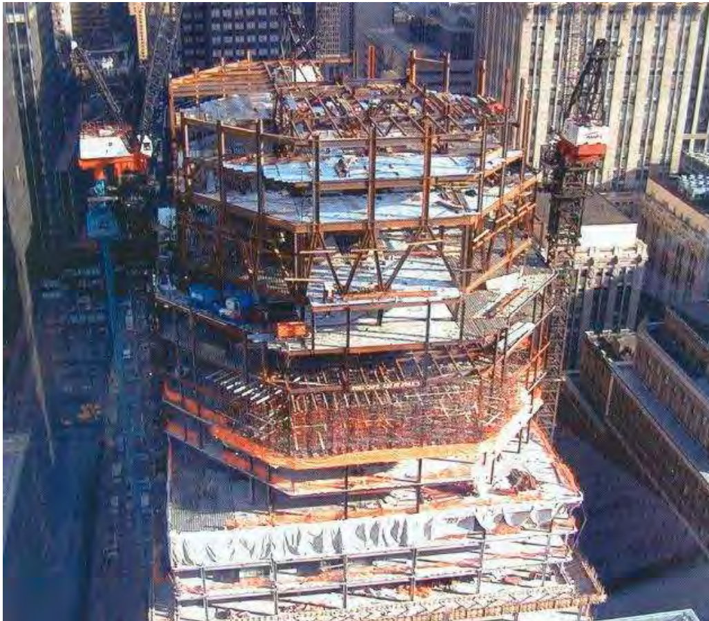
A braced-frame steel structural building in downtown Mahattan.
