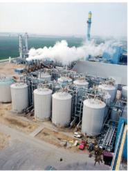
Figure 3 This commercial biogas plant in Texas uses the slurry from 10000 cows as well as other agricultural waste as its raw material
