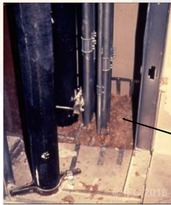
Fire blocking or safing with wool
