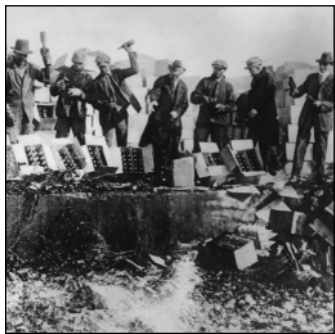
Government officials destroying cases of beer during Prohibition
