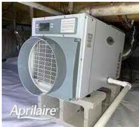
* EXAMPLE ONLY dehumidifier in crawl space
