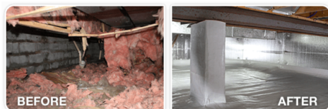
*EXAMPLE ONLY CRAWL SPACE ENCAPSULATION BEFORE AND AFTER
