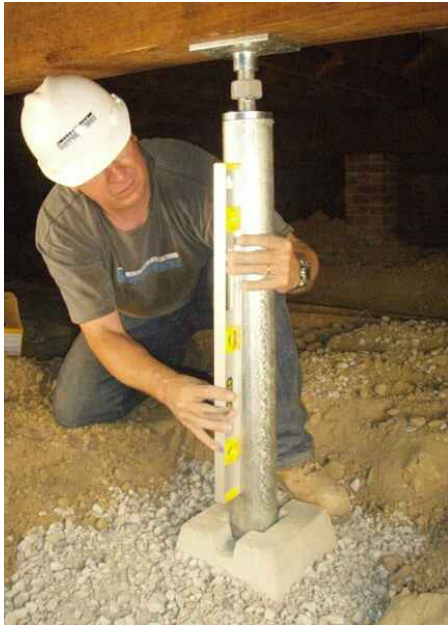
EXAMPLE ONLY REPAIR WITH JACK
