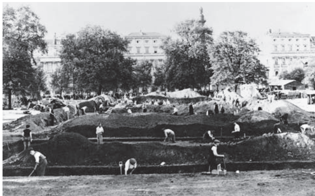
Digging air raid defences in London, September 1938.
