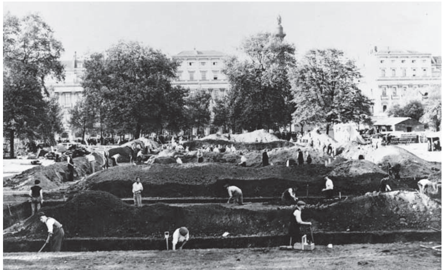
Digging air raid defences in London, September 1938.
