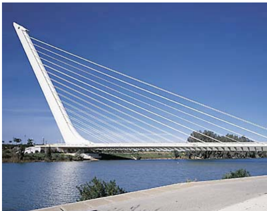
Alamillo Bridge, Spain
