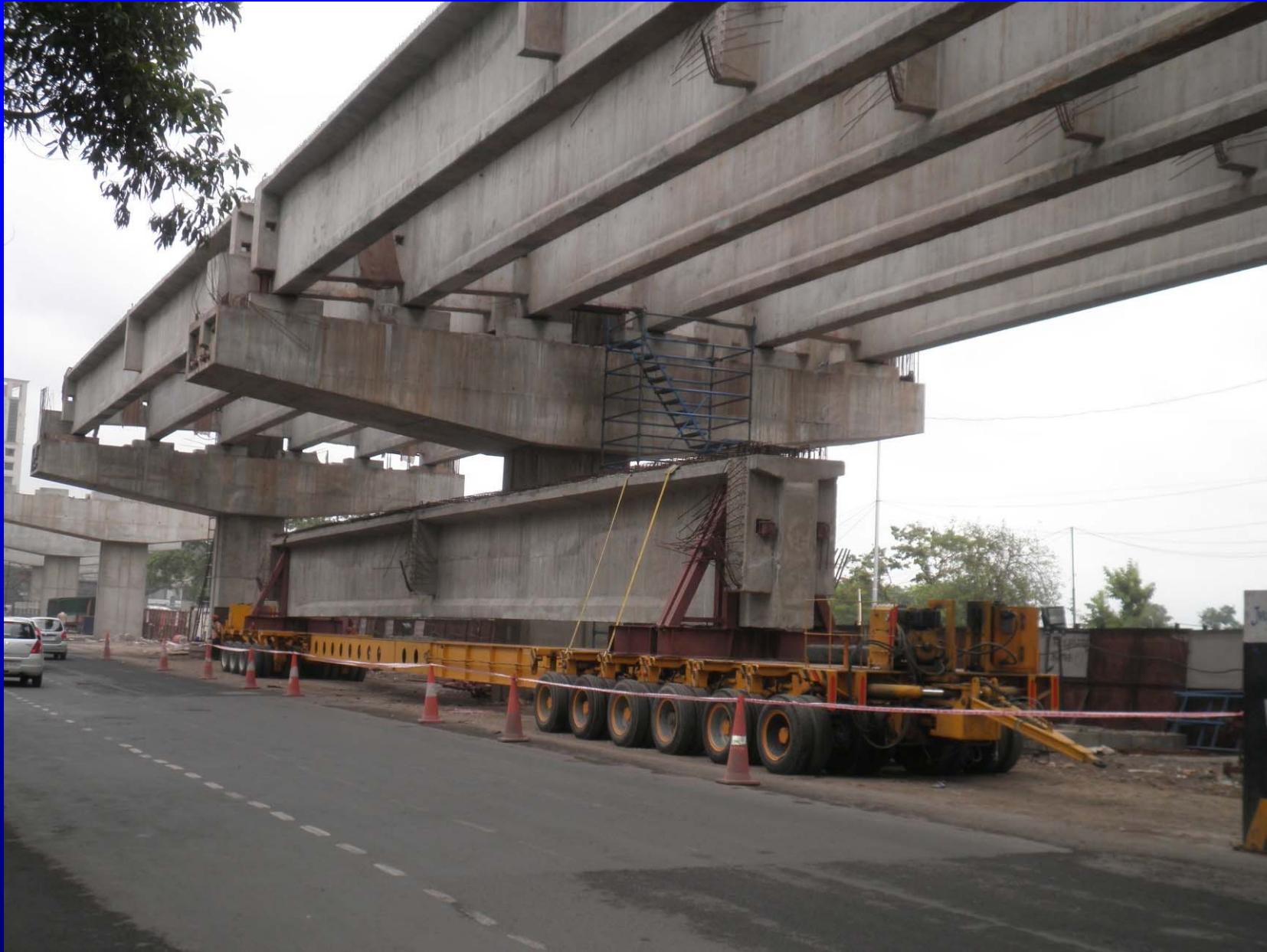
T beam as a bridge girder
