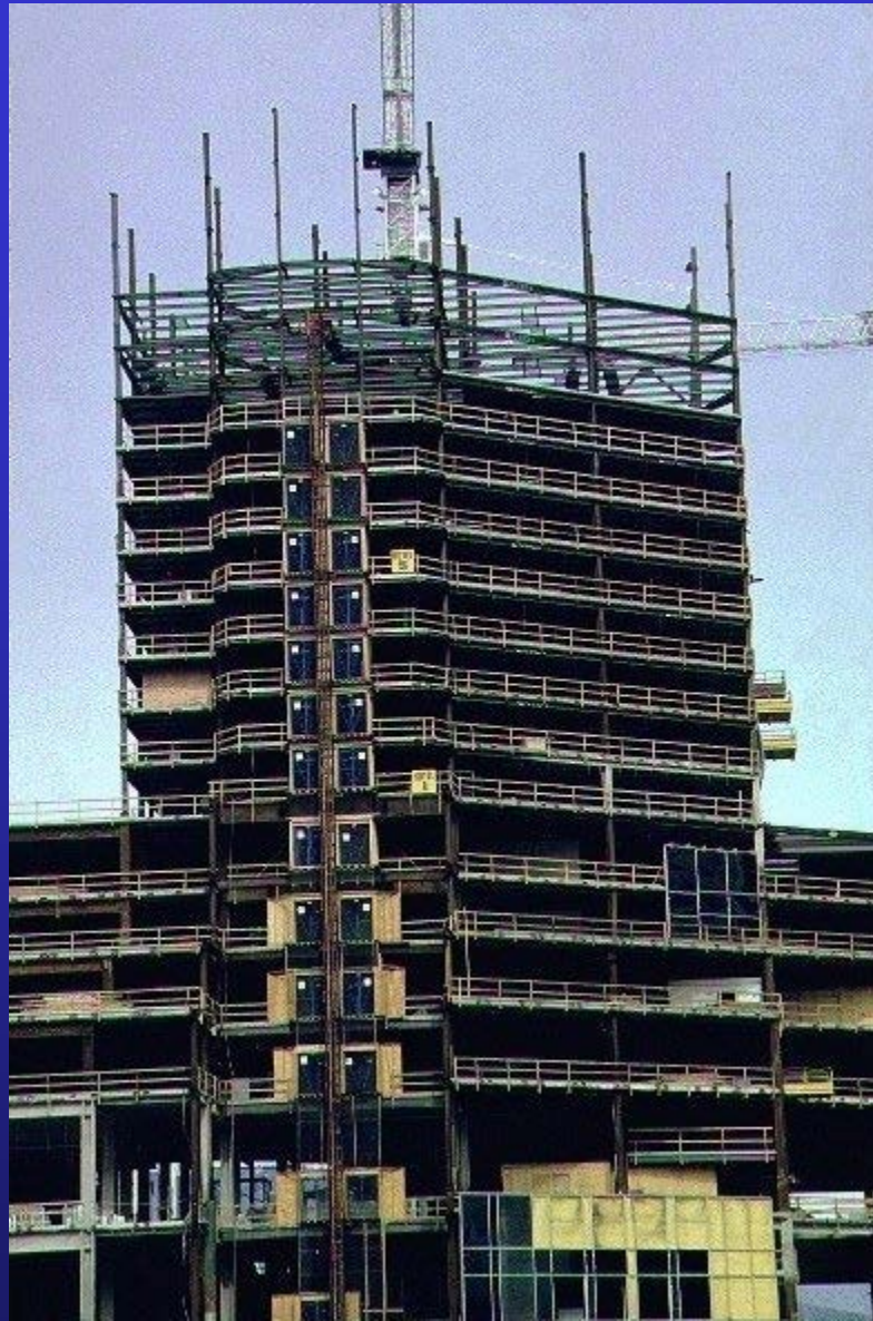
Pan Pacific Hotel and Convention Centre, Vancouver, main tower
