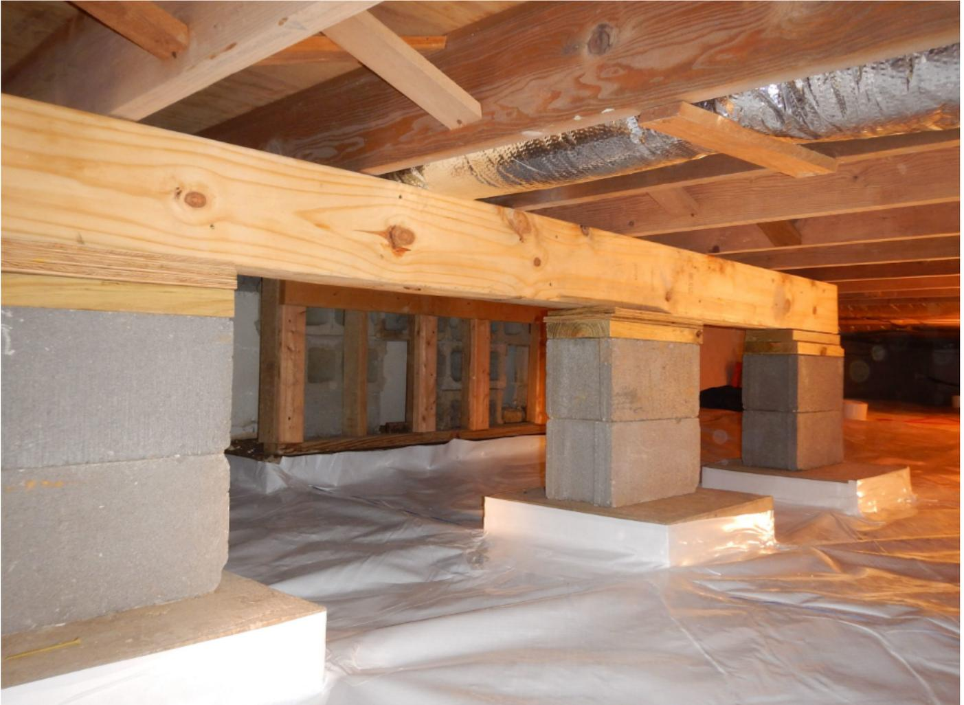
EXAMPLE OF ADDITIONAL PEIRS AND GIRDER BEAMS (CHEAPER OPTION WITH CONCRETE BLOCKS)
