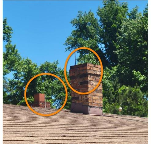
Missing chimney cap observed at the time of inspection.
