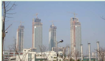
Figure 18 High-rise buildings in Seoul
