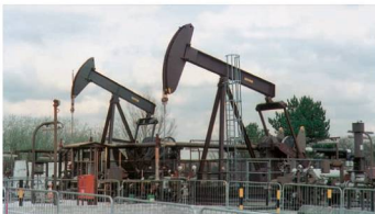
Figure 18 The primary sector: an oil well in Dorset, UK
