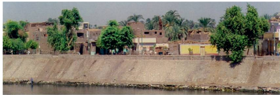
Figure 8 Low-income housing on the banks of the river Nile, Egypt
