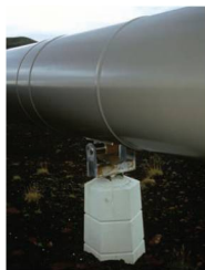
Figure 14 Pipeline on rollers
