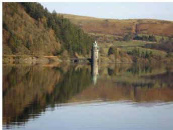
Reservoir with water tower in Wales
