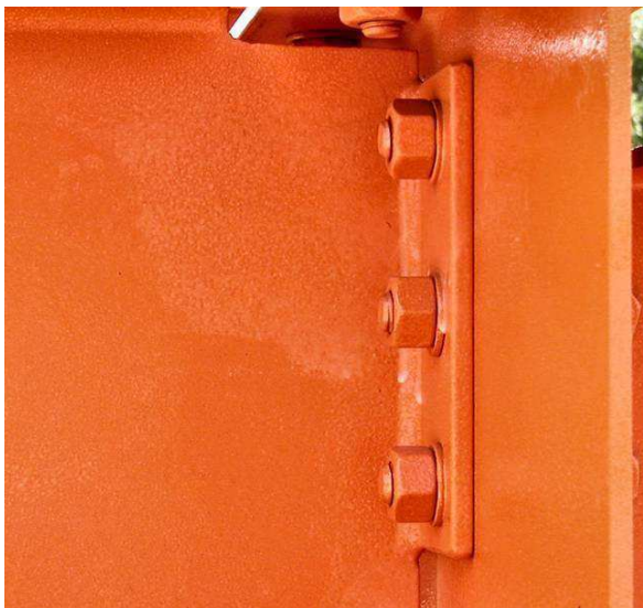
Shear End Plate Connection
