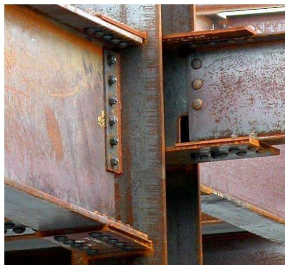
Bolted Flange Plate Connection
