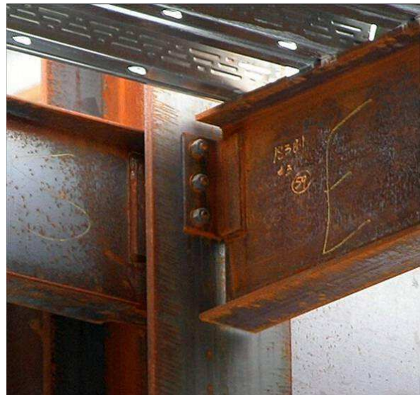
Double Angle Connection
