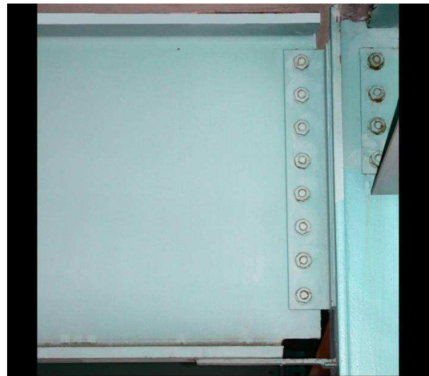
Partially-Restrained (PR) Connections
