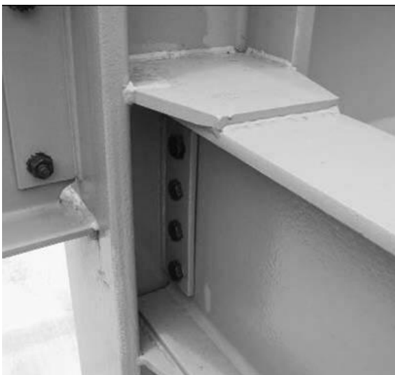
Welded Flange Plate Connection
