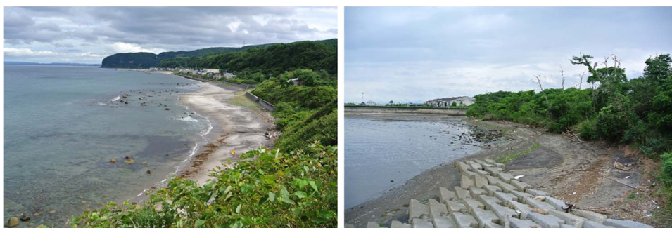
Fig. 3. Kinoppu coast project in Aomori prefecture (left) and Nakatsu Tidal Flat in Oita Prefecture (right) (Photos taken by Naoya Furuta).
