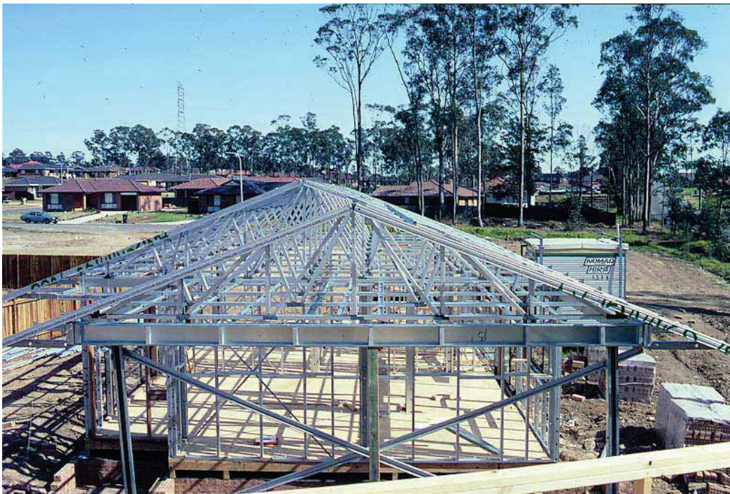
Steel Framed House
