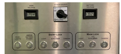
Chamber power panel
