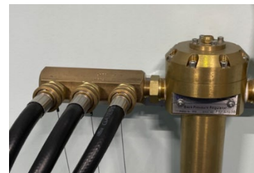
BIBS exhaust ports with back-pressure regulator
