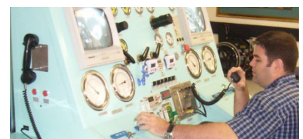
Hyperbaric chamber communications system
