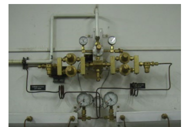
HP oxygen regulator system with change-over
