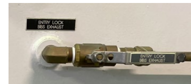
BIBS exhaust shell valve
