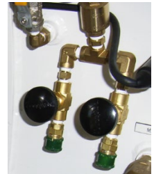
BIBS supply connections
