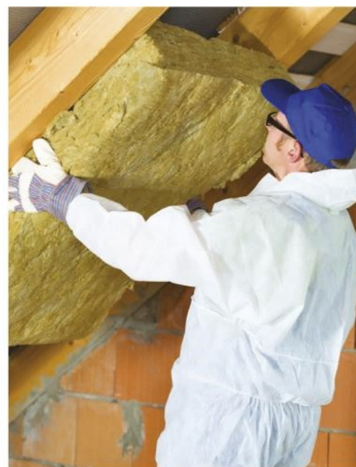
Figure 2 Insulating a loft. The air trapped between fibres makes fibreglass a good insulator
