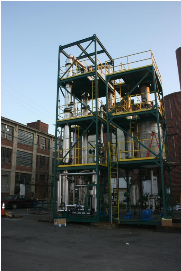
Pacific Biodiesel modules under construction and being shipped
