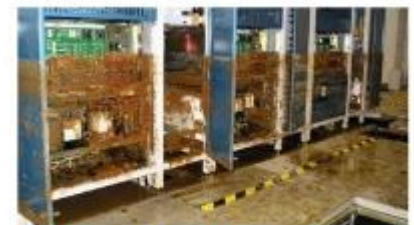
Putting a data center in a basement is a bad idea, in this case drowned DSLAM's
